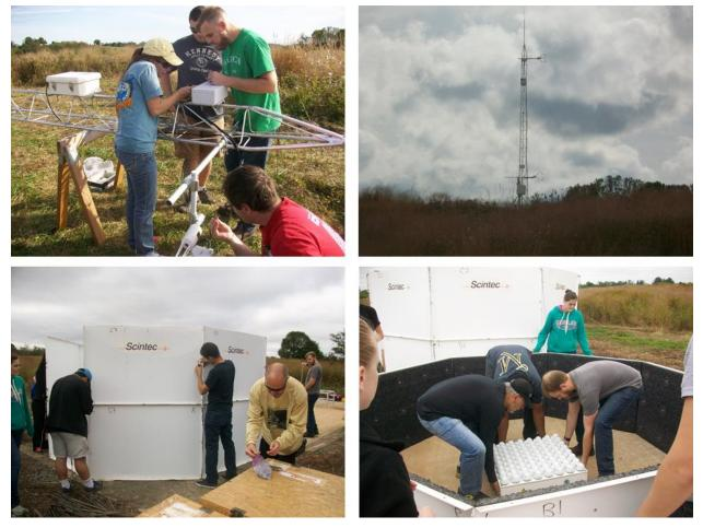
Figure 4: In addition to the UWKA, partner universities deployed a variety of instrumentation. Here is a collage showing Millersville University students installing the flux tower components and assembling the MFAS SoDAR with RASS extension.
