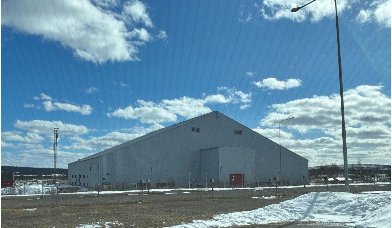
View of the back of the hangar from the parking area. The short posts in the foreground are receptacles to plug in engine block heaters during cold weather.
