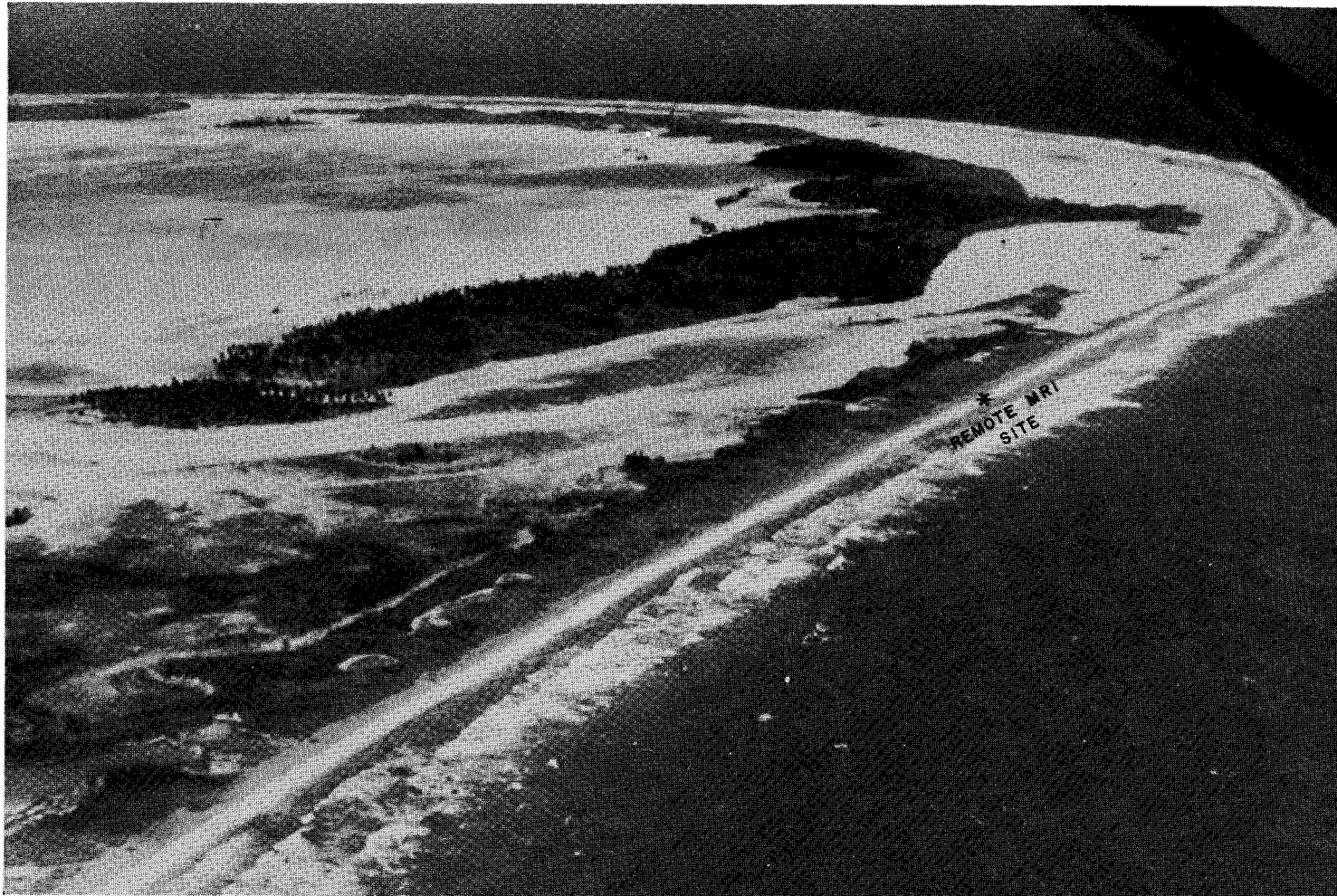
Fig. 17 Aerial view of remote MRI site on western end of Robitaille's Beach, Fanning Island. View is looking northeast from an altitude of 1,200 ft. This site was accessible only by boat, plus wading, and offered excellent off-ocean exposure for all winds except those north of 060 degrees. (NCAR photo)
