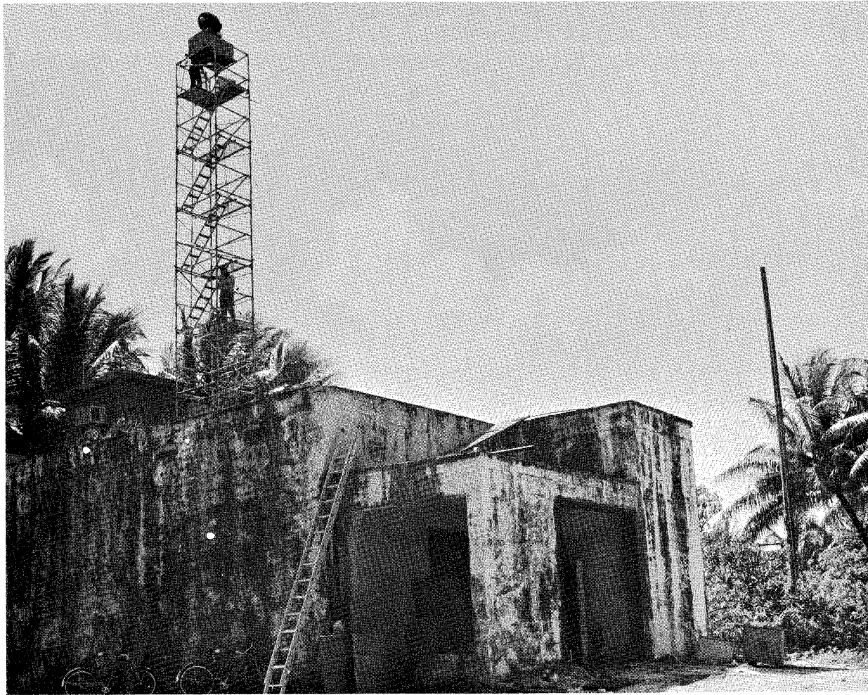
Fig. 10 Radar and photo tower, Palmyra. The antenna is 67 ft above ground level. The photography was carried out from the highest platform on the tower, just below the antenna. The radar equipment is in the air-conditioned shack atop the blockhouse. (NCAR photo)
