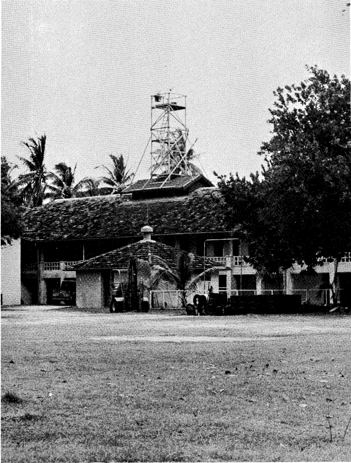
Fig. 19 Photo tower built atop former administration building, Cable Station, Fanning Island. The cameras are elevated 65 ft above the ground. (NCAR photo)
